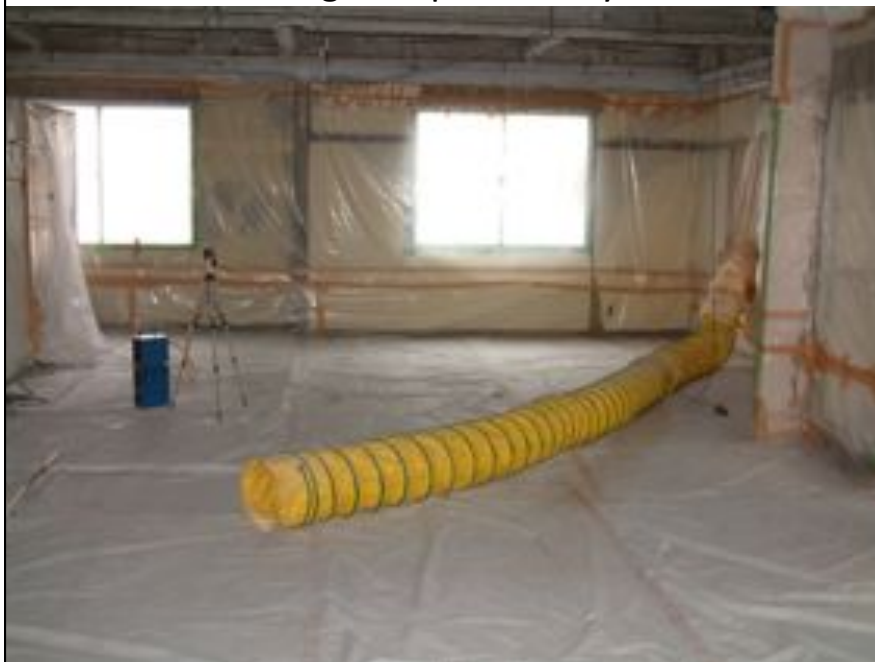
Enclosure and negative pressure system
