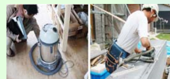
Photo 2 Dust reduction good examples on construction site
